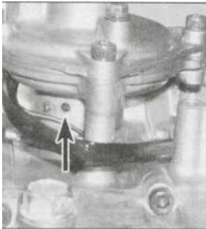
8.2 Check the drain hole (arrowed) for evidence of leakage
