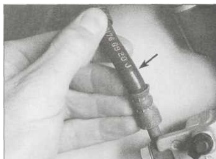
10.2 Flex the brake hoses and check for cracks, bulges and leaking fluid
